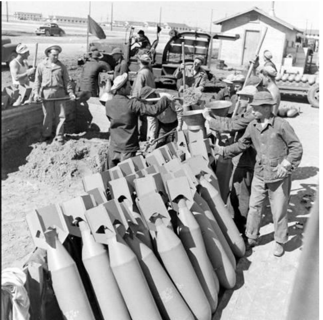
LOADING WITH SAND
