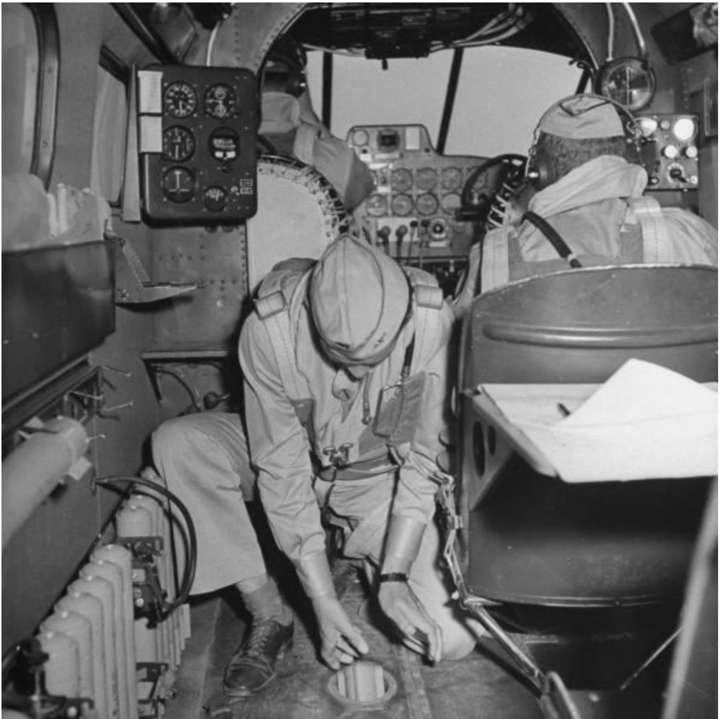
DROPPING SMOKE FLARE TO CHECK DRIFT
